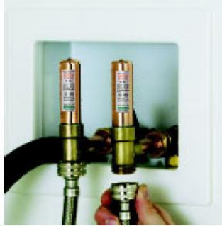
Washing Machine Install between laundry supply valves and hoses
